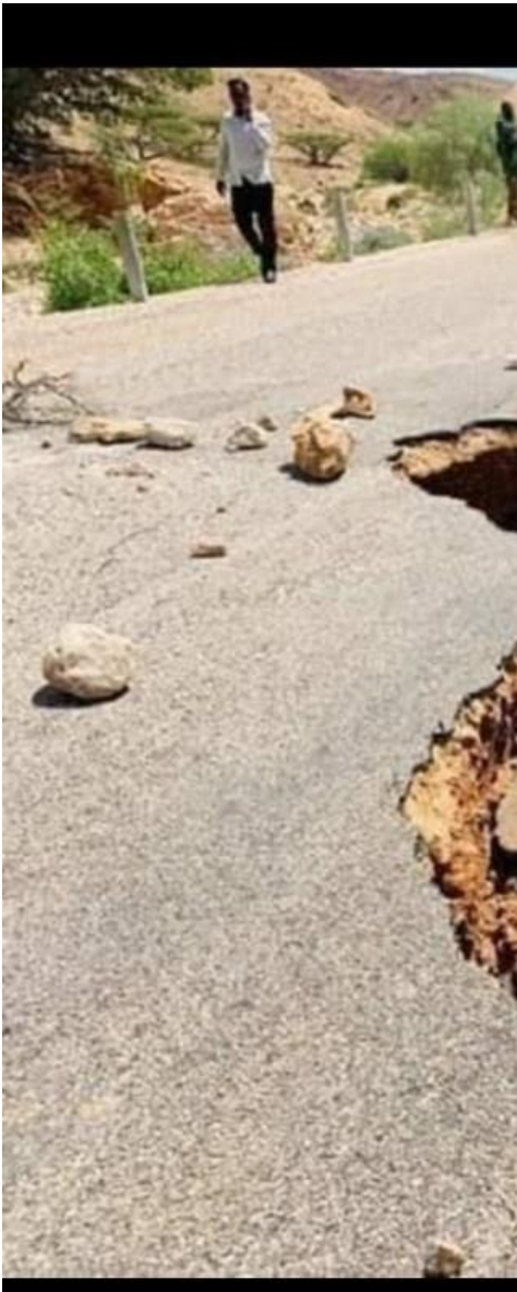
A deep pothole in the Bosaso-Garowe road
