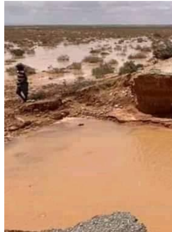
A gully formed in a part of the road between Sunni-jiif and Garowe
