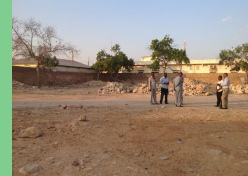
There is a neighbour's boundary wall (beyond) on two edges, fully on one edge, partially on the other.
