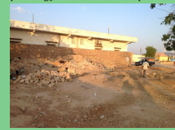
View of existing neighbour's structure (Northeast).
