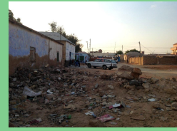
The site will be fenced off and cleared of debris.
