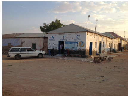
View of adjacent buildings.
