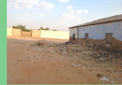
View of neighbour on Southwest.
