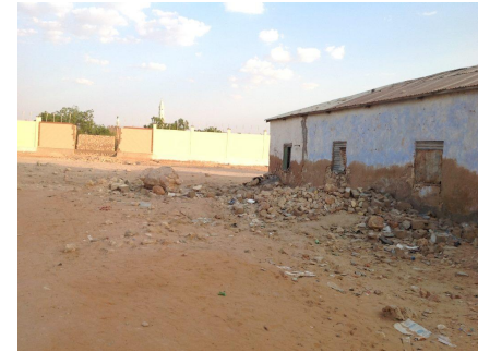
View towards the South of the site.
