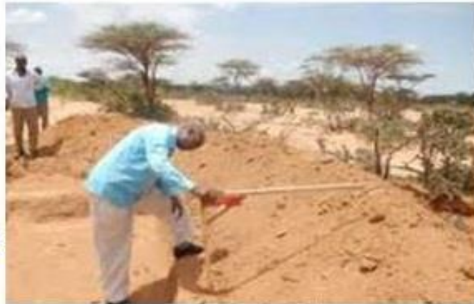
Fig 1. Sankuluh 02 (a), Bocame District, 3D Gullies erosion control structure W=1.2M, L=20M and H=0.8M 130 No. of soil bunds
